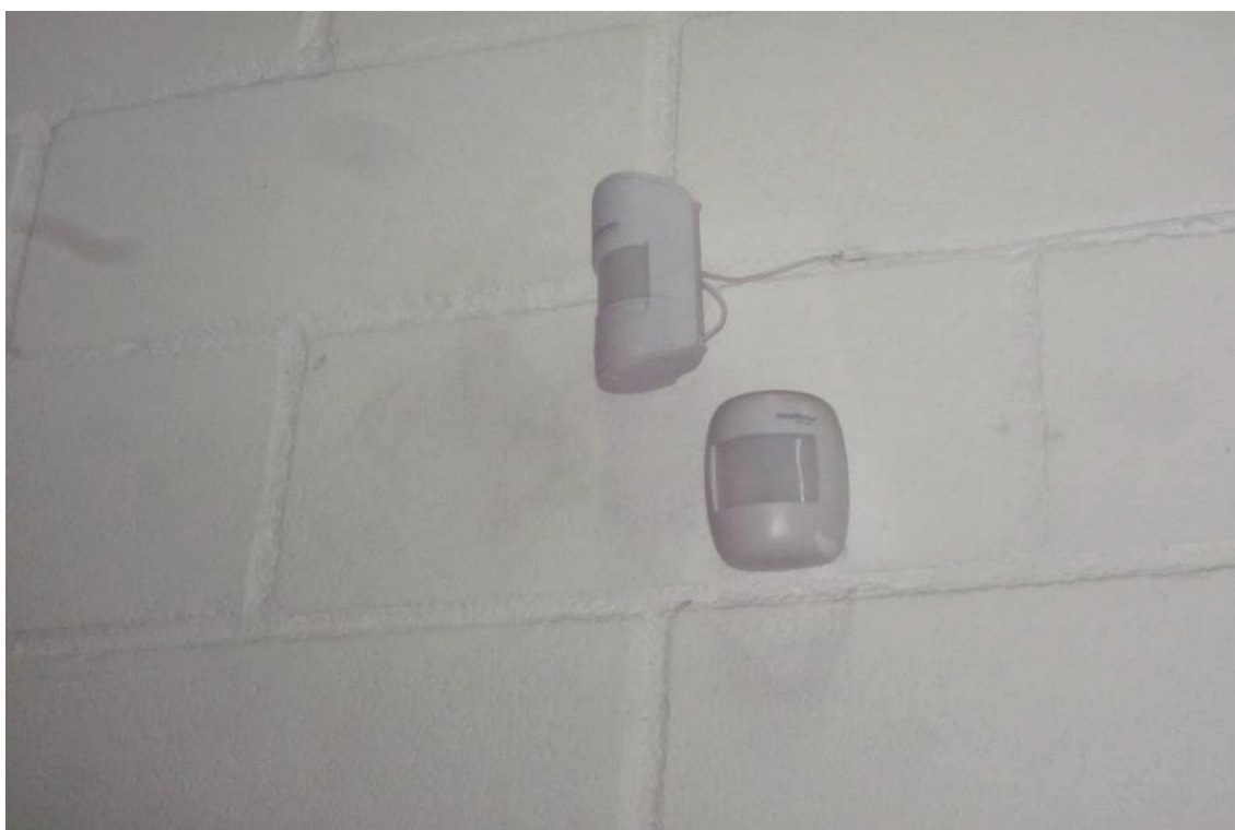
ITENS 1,689 / 1,690 - SENSORES INFRAVERMELHO INTELBRÁS IVP 4101 PET SMART E ECP VISORY RF SAW
